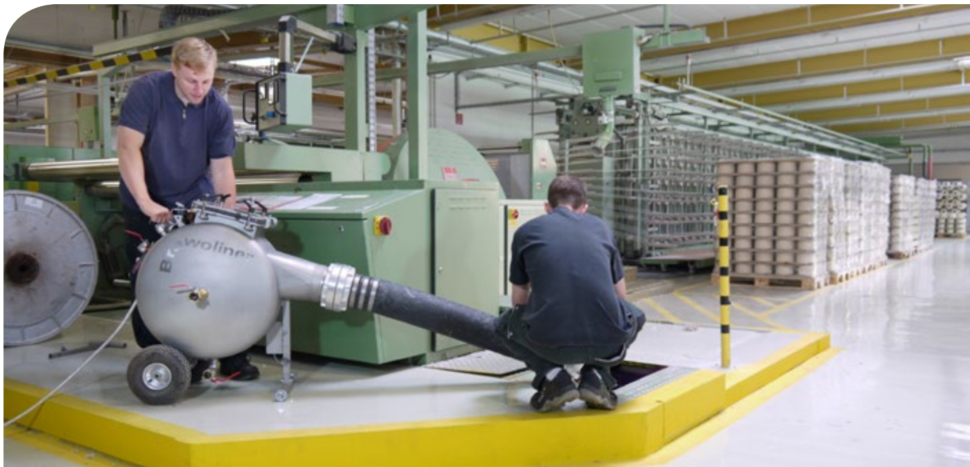
BRAWOLINER® - rehabilitation during production
